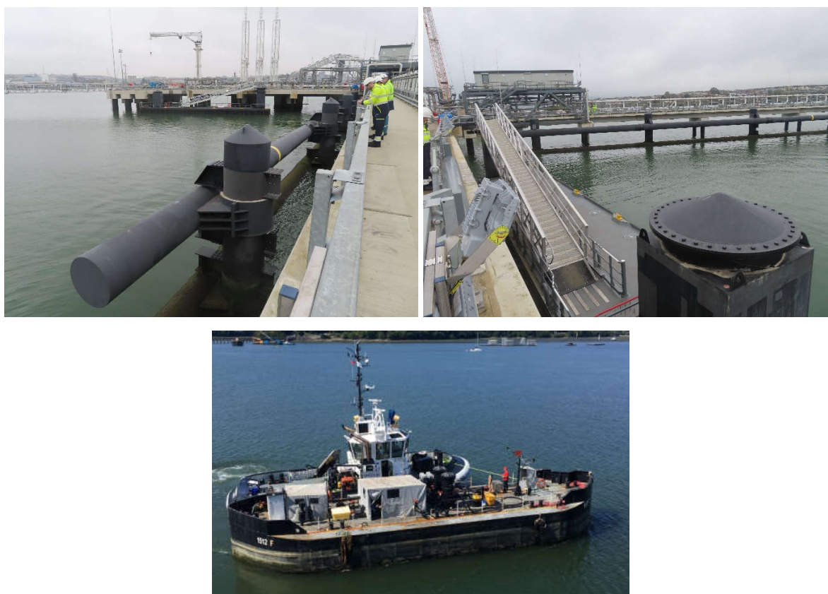
Figure 61: Top: example impact protection installed 2022 at Oil Fuel Depot Thanckes, Dockyard Port Plymouth. Bottom Serco tug towing fuel barge. Source NASH Maritime.
